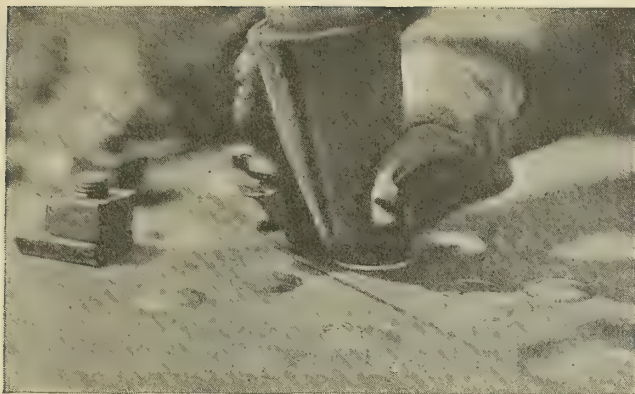
Fig. 19.—Removing Excess Material During Calking Operation
